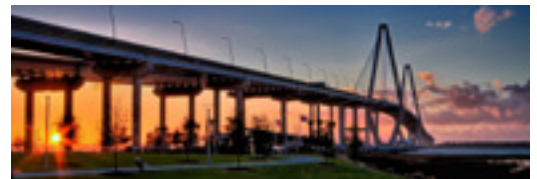
Charleston's famed Cooper River Bridge
